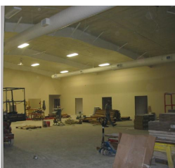
Gym area is painted!
